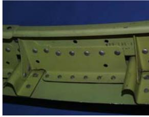
FIG 2. clip-frame-stringer to skin joining
