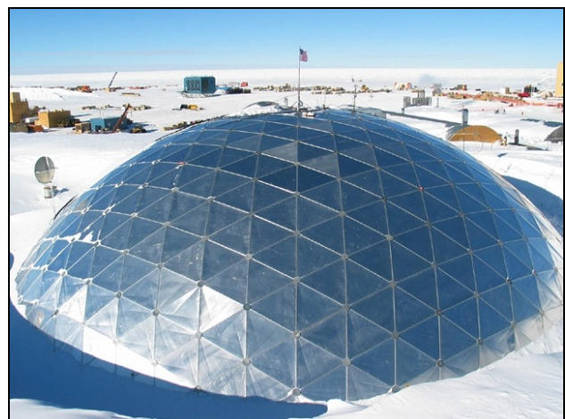
FIG 3. Polar station – geodesic dome, with skin elements
