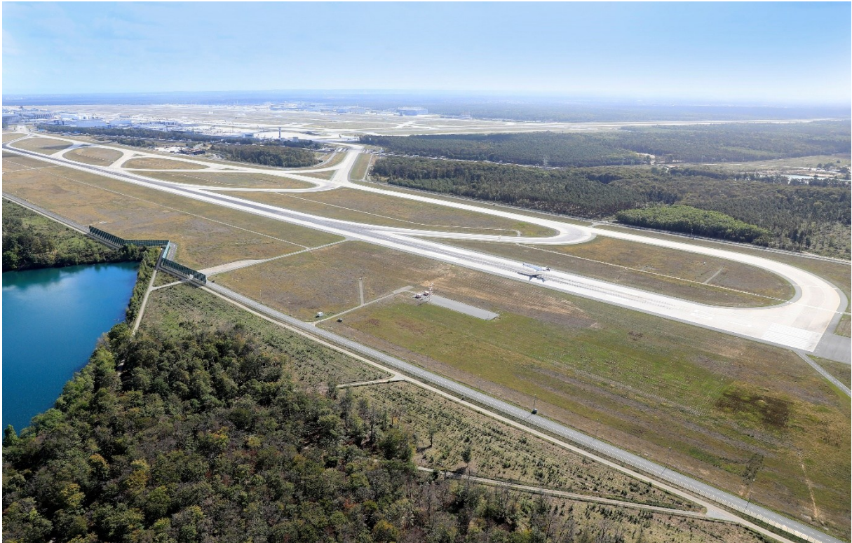
Figure 5.2 Northwest Runway at Frankfurt Airport. Much land, but little available for PV. Photo: Fraport AG. Source: Fraport AG, https://www.fraport.com/en/newsroom/press-releases/2021/q2-2021/frankfurt-airport-to-reopen-northwest-runway-from-june-1.html , https://perma.cc/2ZVP-HBFE .
