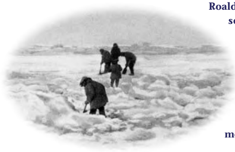
Levelling the ice field to prepare a "runway"
